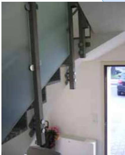
Fixing on stair stringer
