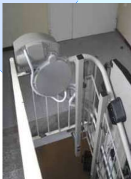
90° drive in the eye of the stair.
