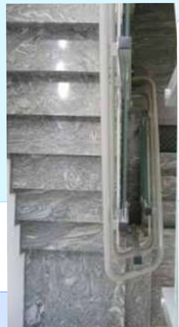
Multi ramps stairs
