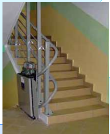
Fixing into the stairwell
